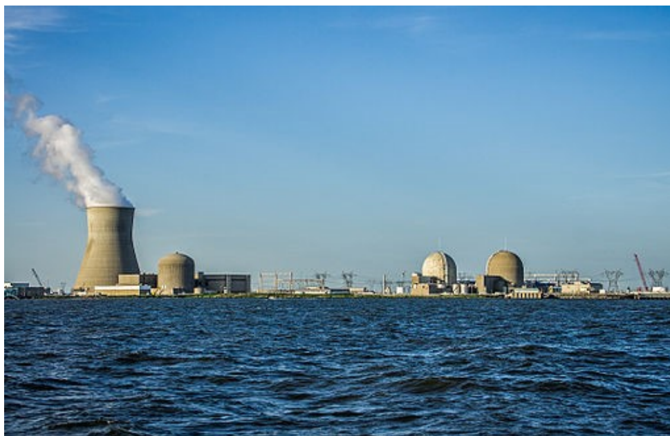
Salem and Hope Creek nuclear reactors
